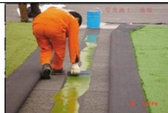
4. Jointing the tape and coating glue on the tape
